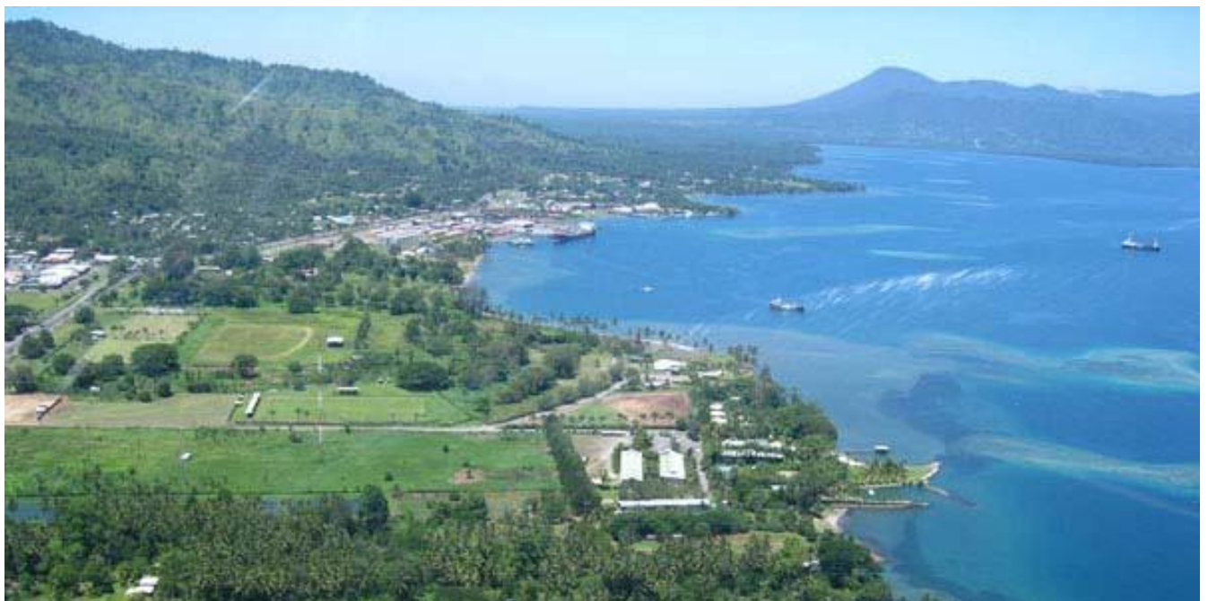
PHOTO 1: Aerial view of the deep water port at the provincial capital of Kimbe
