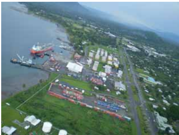
Photo 1: Kimbe Town and Port
